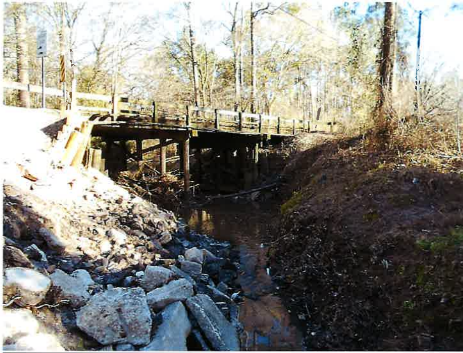
View of upstream section of existing structure.
