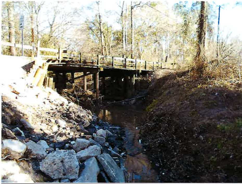
View of upstream section of existing structure.
