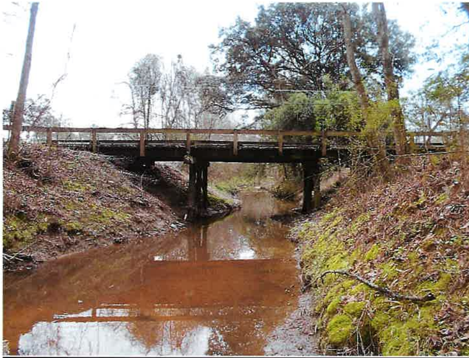
View of upstream section of existing structure.
