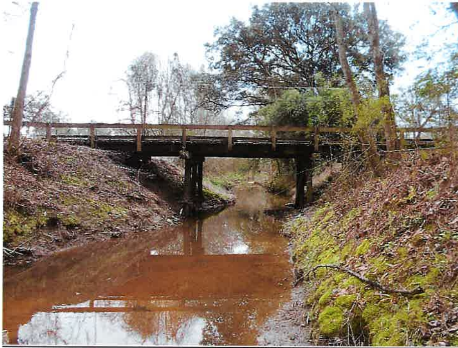
View of upstream section of existing structure.
